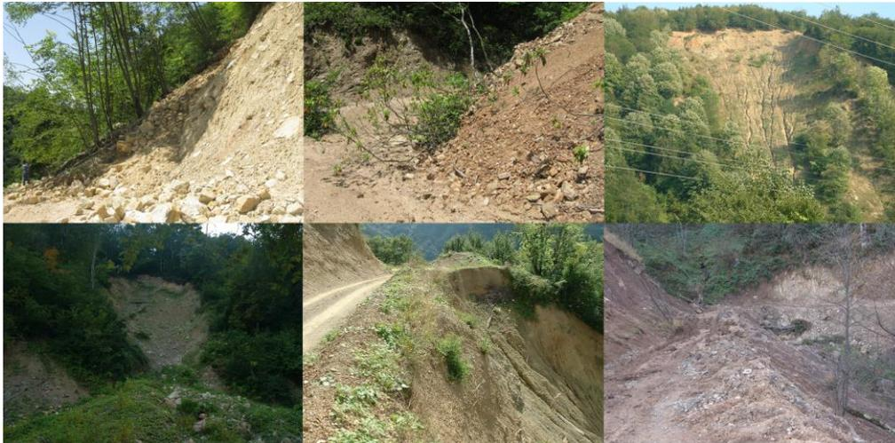
Figure 1. Forest roads damaged by landslides
