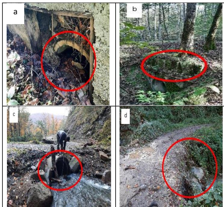
Figure 7. Various failures in pipes across the investigated roads, a, b, c) Intel cracking of pips, d) culvert with the destroyed outlet
