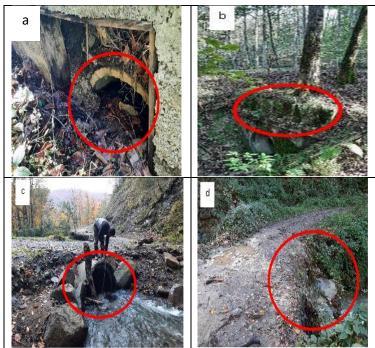
Figure 7. Various failures in pipes across the investigated roads, a, b, c) Intel cracking of pips, d) culvert with the destructed outlet
