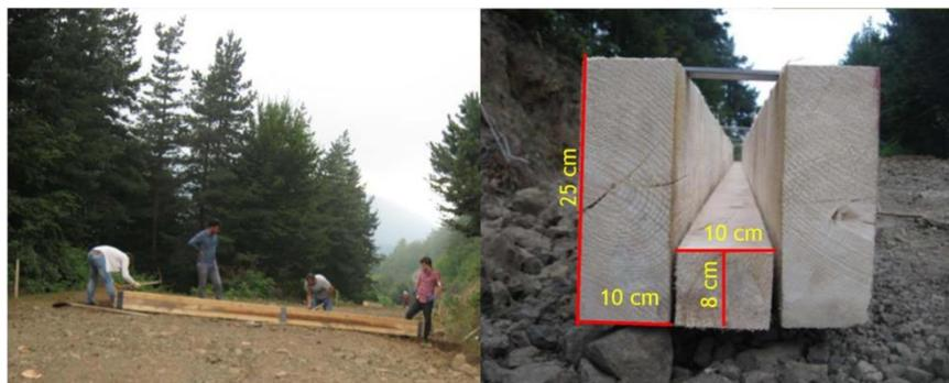
Figure 2. Design of the open-top culverts used in this study
