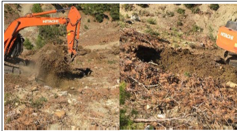
Figure 10. Topsoil excavation after uprooting stump biomass
