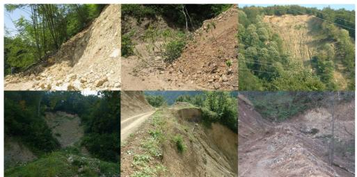
Figure 1. Forest roads damaged by landslides
