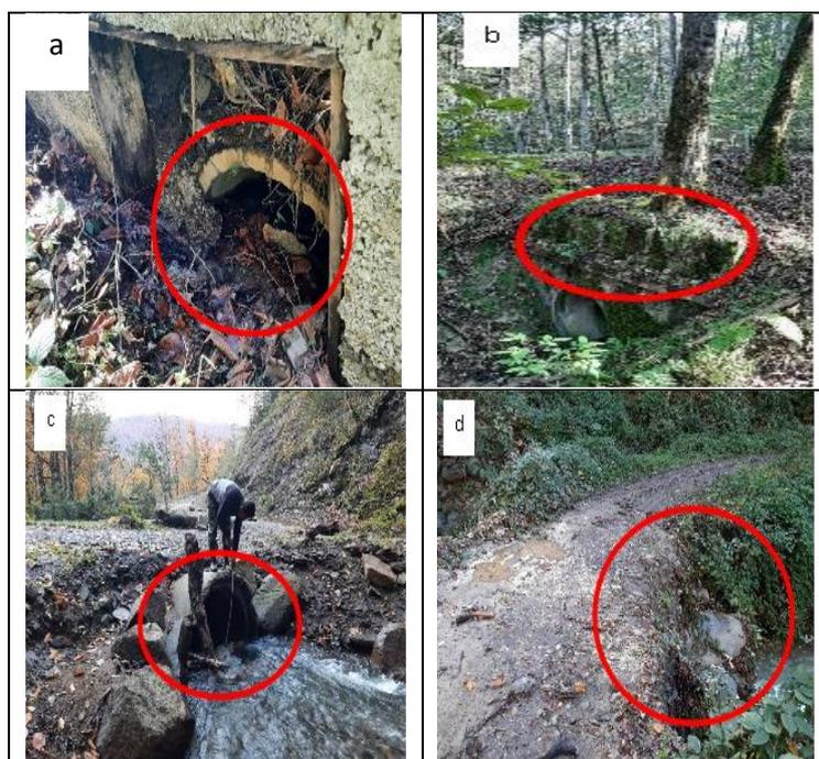
Figure 7. Various failures in pipes across the investigated roads, a, b, c) Intel cracking of pips, d) culvert with the destructed outlet
