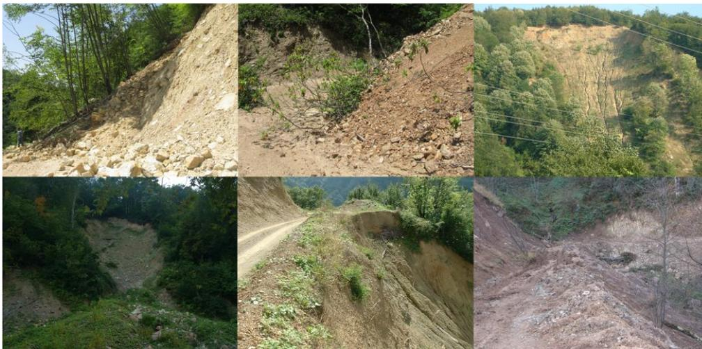
Figure 1. Forest roads damaged by landslides
