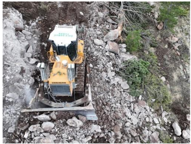
Figure 15. Shovelling with dozer
