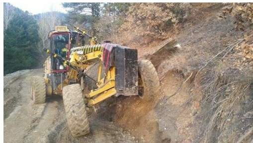
Figure 19. Leveling excavation slopes with a grader
