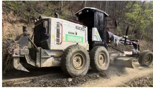
Figure 20. Surfacing and shaping for road platform
