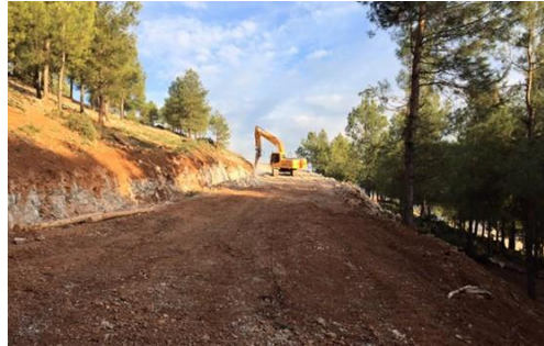
Figure 21. Ditch forming with excavator after road surfacing
