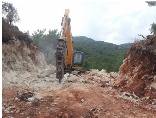
Figure 16. Smoothing with excavator for subgrade design
