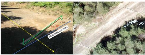
Figure 3. The open-top culverts are installed over the road surface
