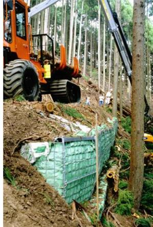
Figure 2. Retaining wall (L-shaped steel retaining wall) utilizing road width efficiently
