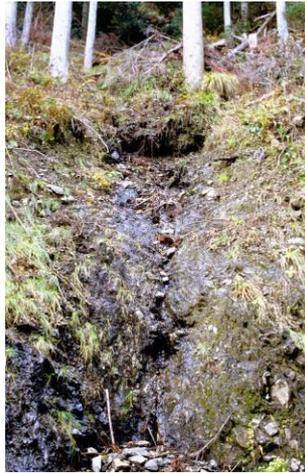
Figure 5. An example of crushing zone and welling water where L-shaped mesh wall was prescribed
