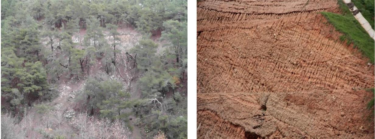
Figure 1. Damage caused by forest road construction on steep slope grades
