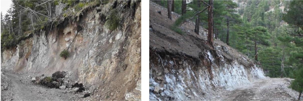
Figure 4. Material fall and trees with broken stability on newly build roads
