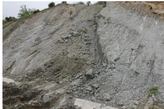
Figure 3. During snow fighting, degradation of road slope and landslides on new formed slopes.
